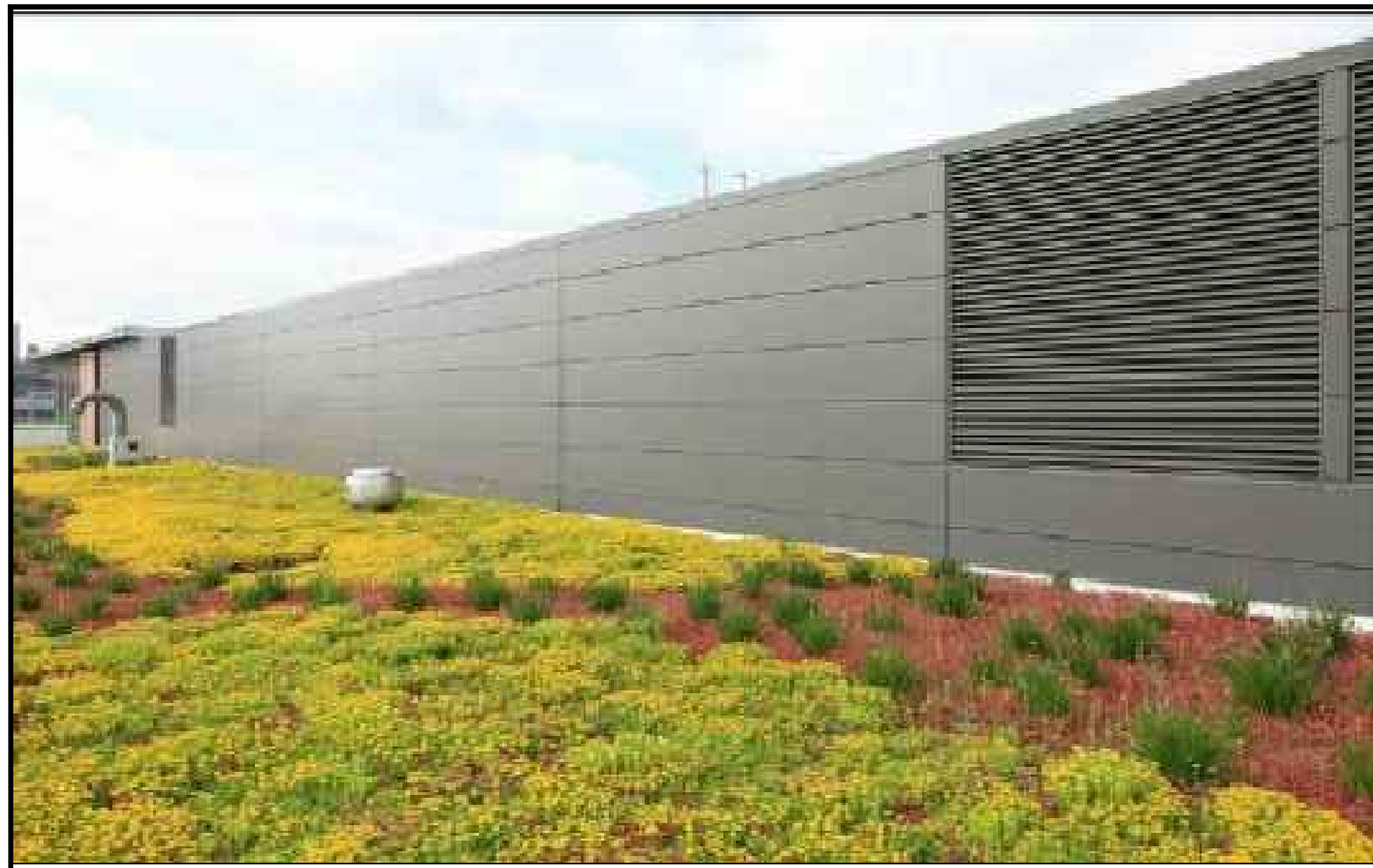
A. GREEN ROOF
